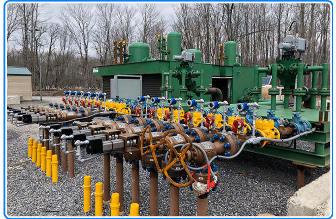
Seneca's twelve flowlines connect individual wells from the wellhead and bulk test units.
