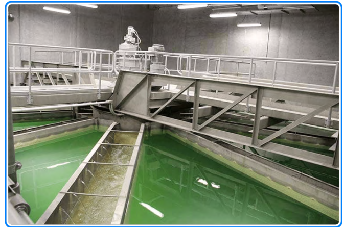
Contact basin where water coming in is being mixed with lime and chemicals for softening and to settle out the solids.
