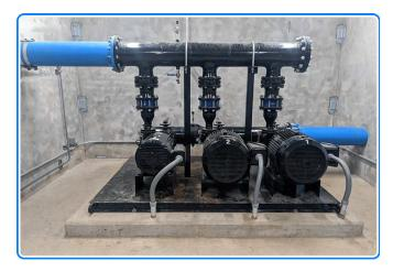
This is one of 15 pump stations throughout the city that collects sewage or wastewater and stores it in a chamber. The collection is an intricately designed system that uses a series of downstream pipes, pumps, and controls. Helping ensure this series of complex processes works properly and keeps wastewater from entering Lake Granbury is SmartSights remote alarm notification software.
