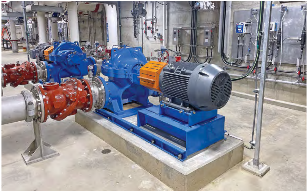
Figure 1. The new water treatment plant has a raw water pump station that pumps water from Comox Lake.
