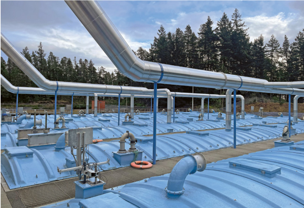
Figure 2. The Comox Valley Regional District's bioreactors are just one of the many pieces of equipment its SCADA system monitors.
