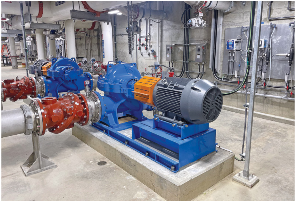
Figure 1. The new water treatment plant has a raw water pump station that pumps water from Comox Lake.
